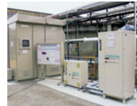
A pilot plant that supplies hydrogen manufactured by an electrolytic plant directly to fuel cells through the pipeline
