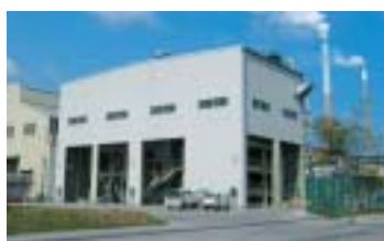
No. 4 unit at the waste plastic crushing facility
