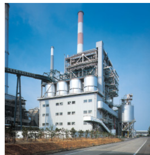
Private power generation plant with one of the largest generating capacities in Japan
