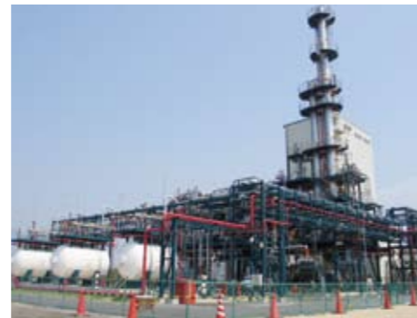
Verification plant for manufacturing polycrystalline silicon for solar cells
