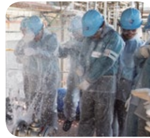
Getting sprayed by a leaky pipe
