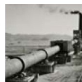
1960's Cement kiln (length: 185m)
