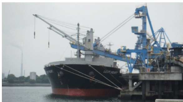
Clinker ship loader (Tokuyama Factory)
