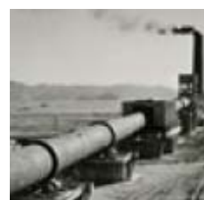
1960's Cement kiln (length: 185m)
