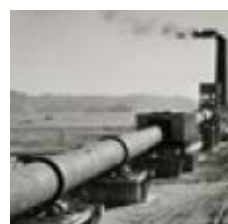
1960's Cement kiln (length: 185m)
