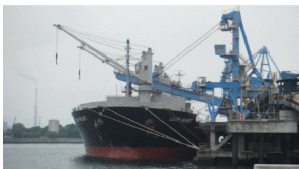
Clinker ship loader (Tokuyama Factory)
