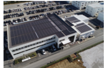
Kashima Factory building with solar panels installed
