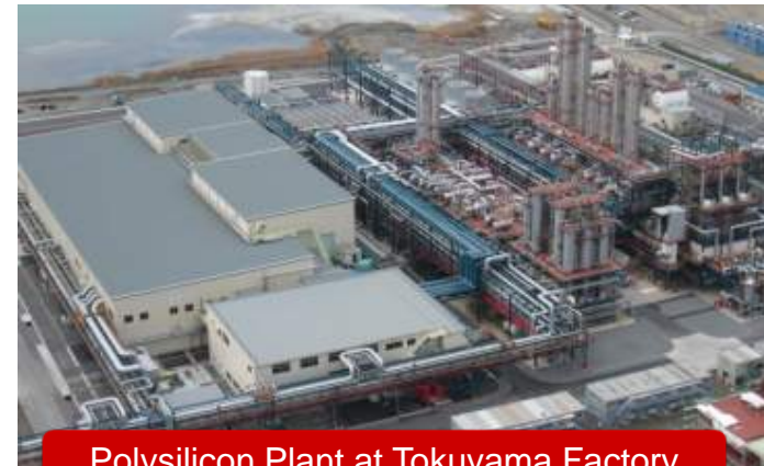
Polysilicon Plant at Tokuyama Factory
