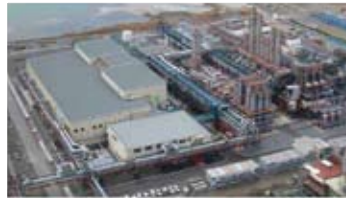
Polycrystalline silicon plant at the Tokuyama Factory
