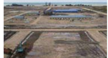
Construction site at the Samalaju Industrial Park
