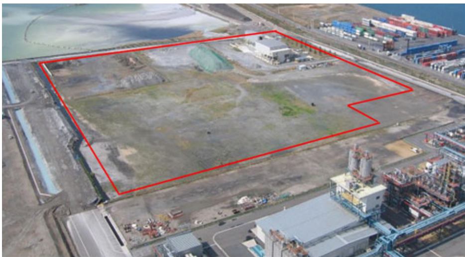
Building site at Higashi Plant
