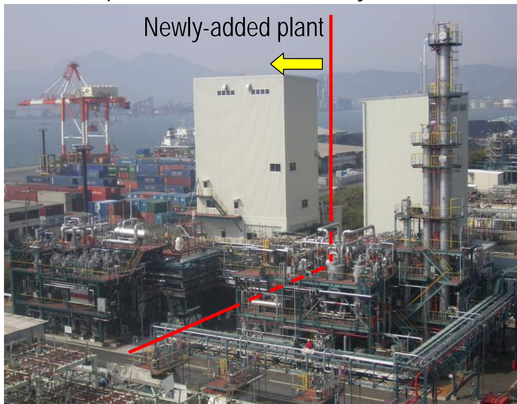
VLD verification plant
