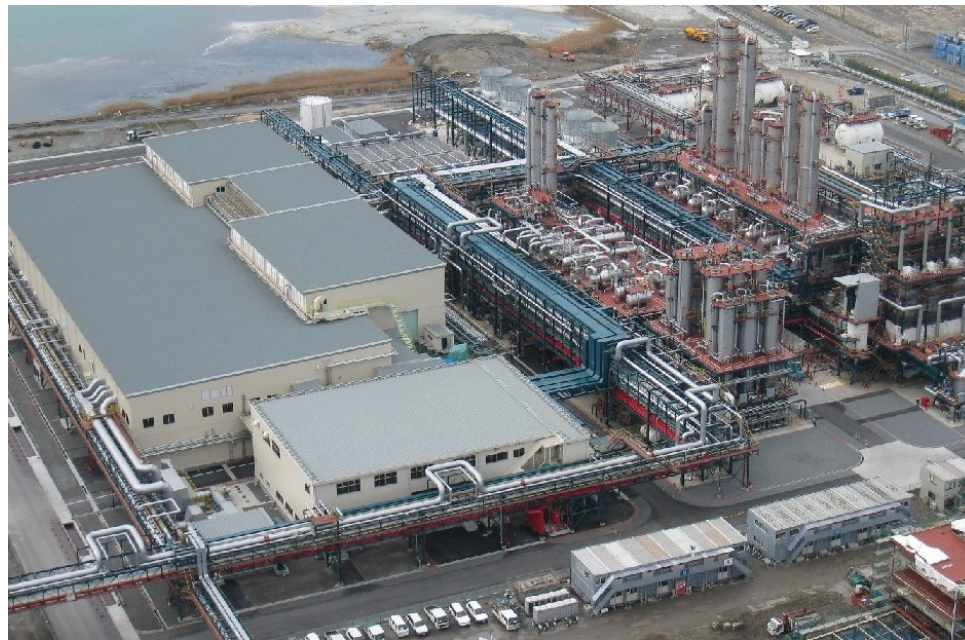
Polysilicon plant completed (Higashi Plant)
