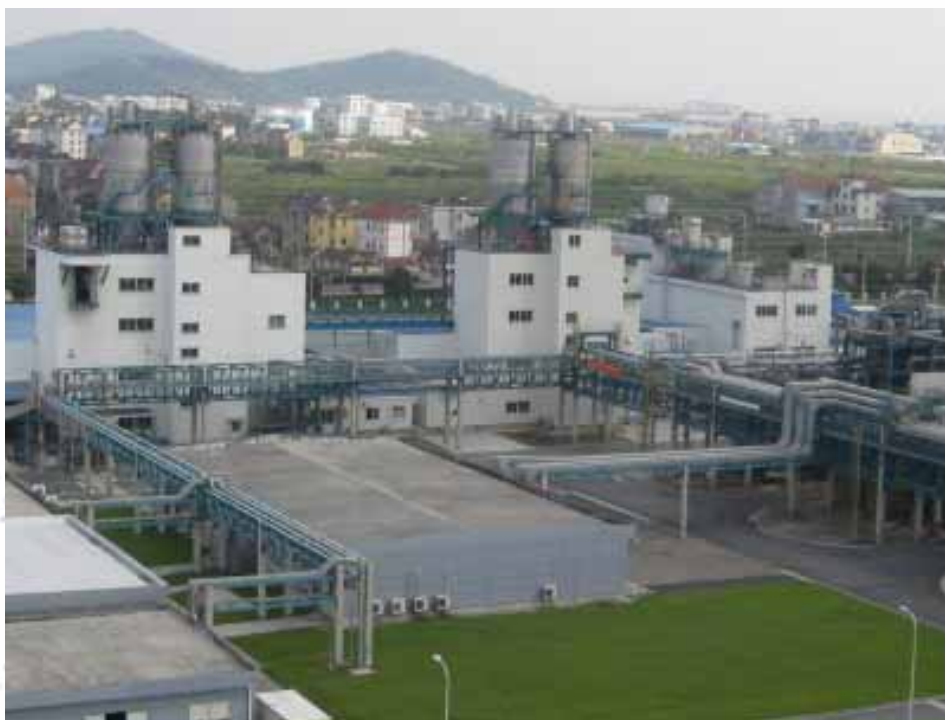
The 2nd phase facilities that is complete (on the right)
