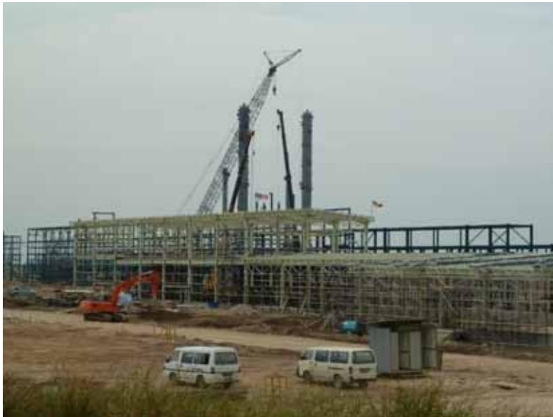
The 1st-phase plant construction in progress
