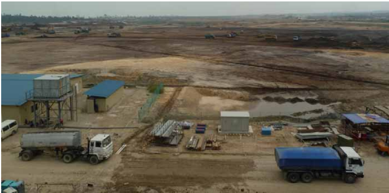
Preparation of the ground for the 2nd-phase plant construction
