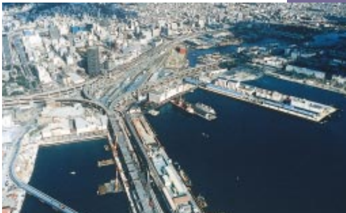
Reconstruction continues apace in earthquake-ravaged Kobe.
