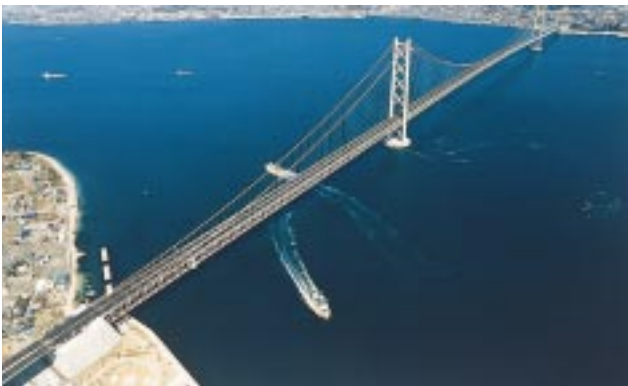
Tokuyama's high-flowability, low-heat cement was used to anchor the Akashi Kaikyo Bridge.
