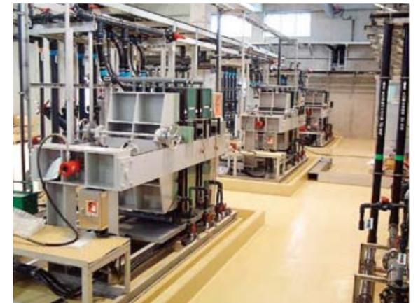
The *ACILYZER* high-performance electrolysizer based on ion exchange membranes
