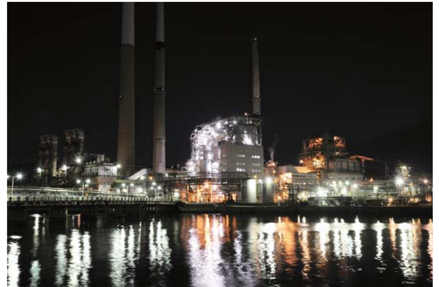
View of the central power plant from the Nanyo Plant
