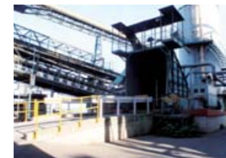
High-moisture sludge facilities
