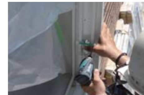
Installation of fire-resistant parts
