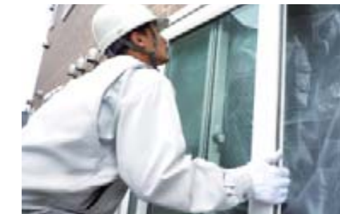
Replacement of plastic window sashes
