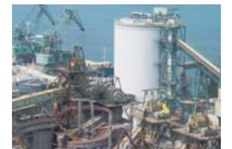
Coal ash facilities
