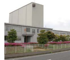
Location: 3075-18 Shimasu, Itako-shi, Ibaraki, Japan Number of employees: 197 Total site area: 89,800m 2
