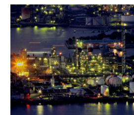
Location: 1-1 Harumi-cho, Shunan-shi, Yamaguchi, Japan Number of employees: 63 Total site area: 70,997m 2
