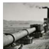
1960's Cement kiln (length: 185m)
