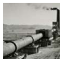
1960's Cement kiln (length: 185m)
