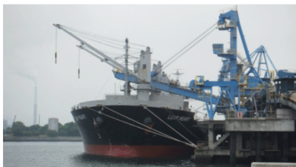
Clinker ship loader (Tokuyama Factory)
