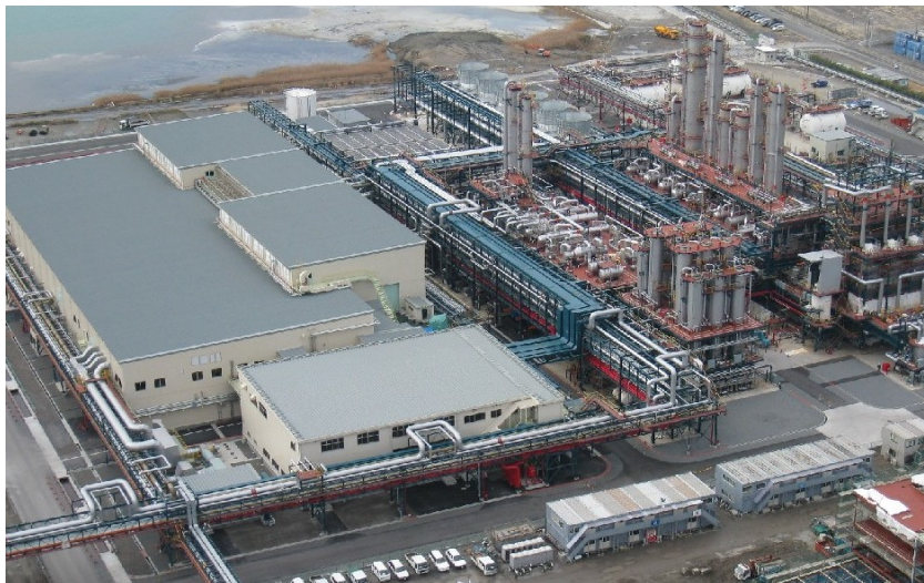
3,000 ton plant started commercial operations in April 2009 (Tokuyama Factory's Higashi Plant)
